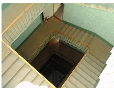
Escalier principal Phot. François Fouger IVR82_20057300785NUCA
