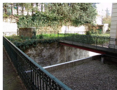
Passerelles Phot. François Fouger IVR82_20057300787NUCA
