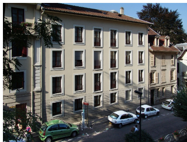
Façade orientale Phot. François Fouger IVR82_20047300525NUCA
