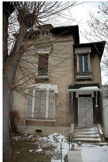
Elévation principale Phot. Maryannick Chalabi IVR82_20066900644NUCA
