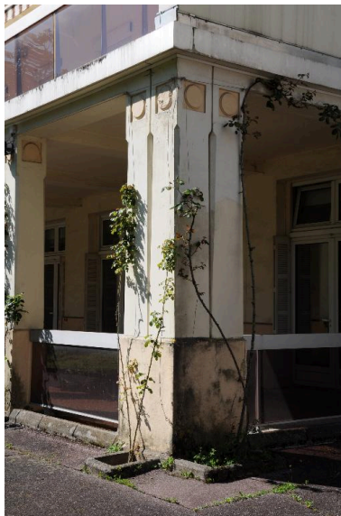
Pilier supportant la terrasse Phot. Denys Harreau IVR82_20147300543NUCA
