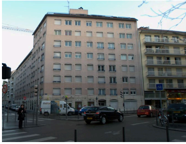
Elévation principale Phot. Maryannick Chalabi IVR82_20116904083NUCA
