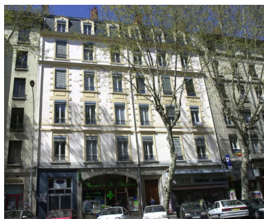
Elévation principale Phot. Maryannick Chalabi IVR82_20036900362NUCA
