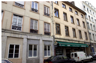
Elévation rue Denuzière Phot. Maryannick Chalabi IVR82_20016902106NUCA
