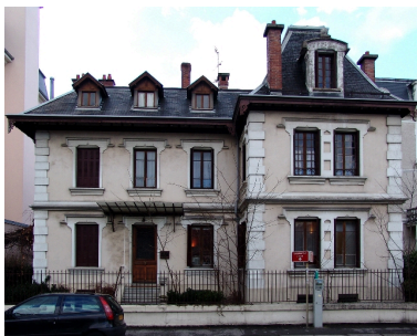
Façade principale Phot. François Fouger IVR82_20057300124NUCA
