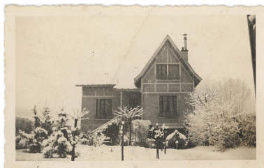
Façade nord. Photograph. milieu XXe siècle Repro. Philippe Gras IVR84_20177300463NUCB
