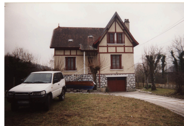
Façade nord. Photograph. 2002 Repro. Philippe Gras IVR84_20177300464NUCB
