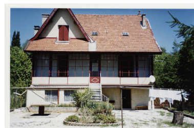
Façade postérieure. Photograph. 2003 Repro. Philippe Gras IVR84_20177300467NUCB
