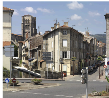
Vue de situation. Phot. Didier Gourbin IVR82_20064202567NUCA
