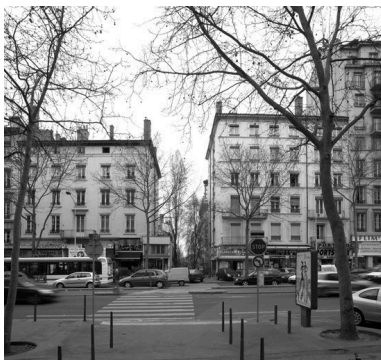
Elévation principale Phot. Eric Dessert IVR82_20056900655NUC
