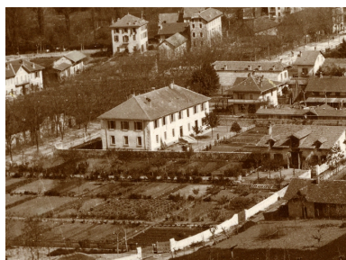
Façade orientale Repro. François Fouger IVR82_20097301029NUCB
