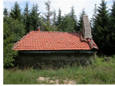
Gouttereau nord-est. Phot. Caroline Guibaud IVR82_20124201477NUCA
