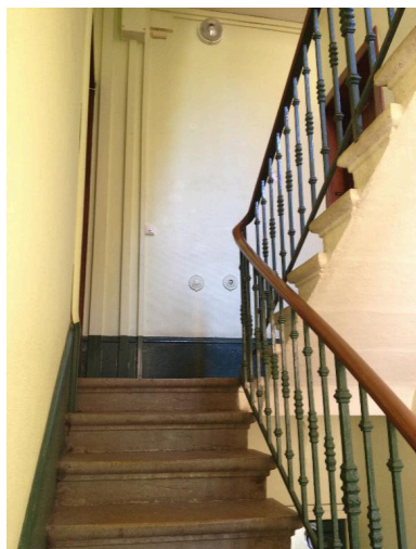
Palier Phot. Noémie Caillat IVR82_20156900603NUCA
