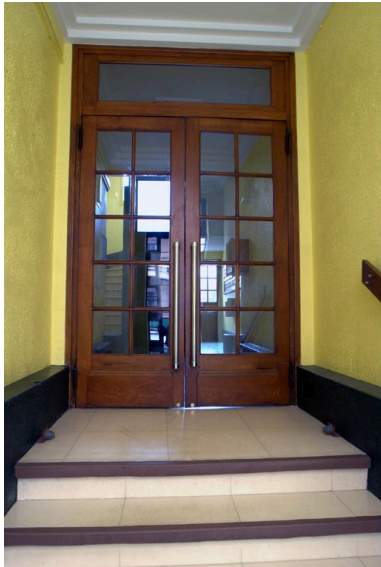
Vestibule, sas Phot. Maryannick Chalabi IVR82_20106903580NUCA
