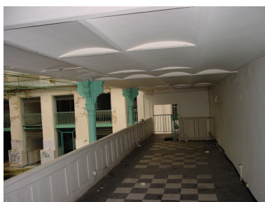
circulation haute Phot. Philippe Marin-Lafèche IVR82_20086900325NUCA
