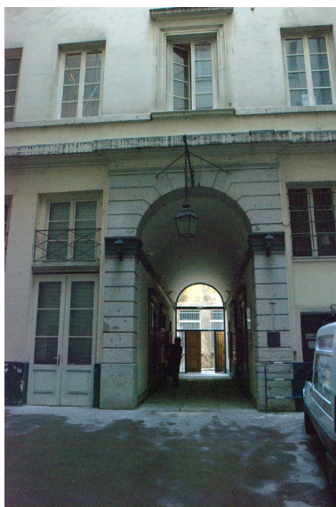
Cour traversante Phot. Nadine Halitim-Dubois IVR82_20086900236NUCA
