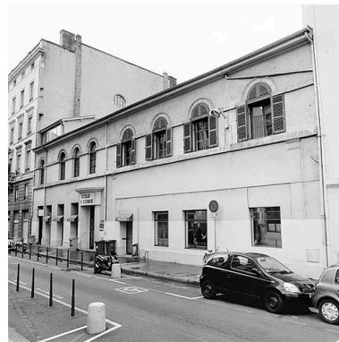
Façade est, rue Vaubecour Phot. Didier Gourbin IVR82_20046902714X
