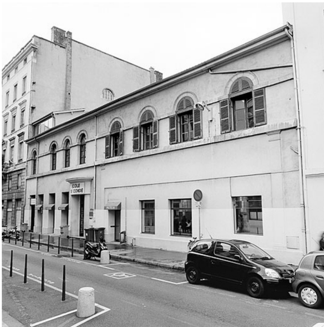
Façade est, rue Vaubecour
