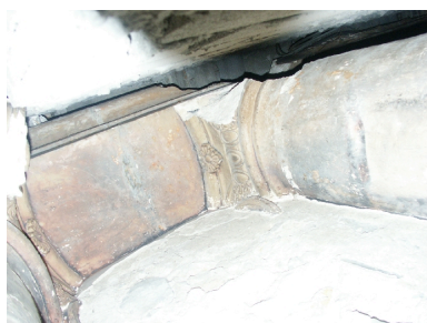
Colonnes avant restauration Phot. François Fouger IVR82_20047300371NUCA
