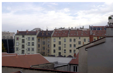
Elévation postérieure Phot. Maryannick Chalabi IVR82_20086900643NUCA
