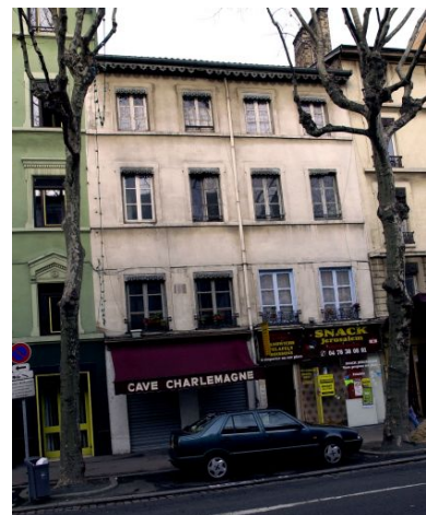
Elévation principale Phot. Maryannick Chalabi IVR82_20016900236NUCA
