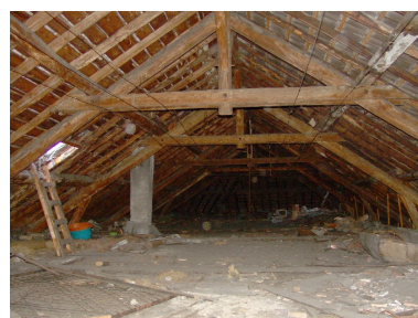
Charpente Phot. François Fouger IVR82_20057300015NUCA
