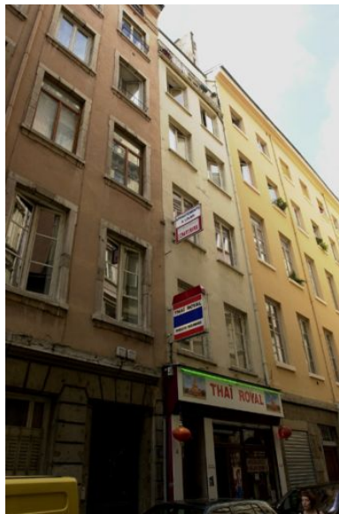
Façade Phot. Bernard Ducouret IVR82_20046900776NUCA
