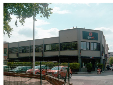
Elevation sur Rue Prosper Chappet Phot. Salohy Rakotomalala IVR82_20106901484NUCA
