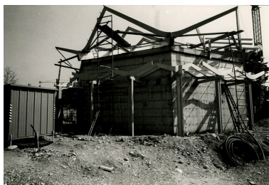
Eglise, pose de la charpente Repro. Maryannick Chalabi IVR82_20096900907NUCA
