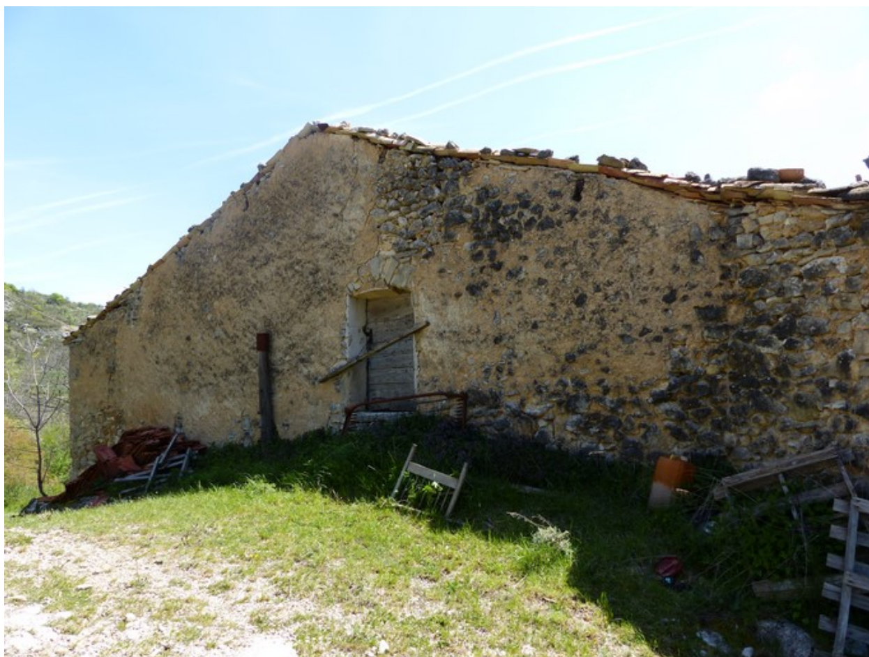
Ensemble oriental. Pignon nord.
