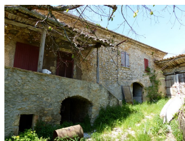
Ensemble occidental. Elévation est. Phot. Alexeï Laurent IVR84_20162600755NUCA
