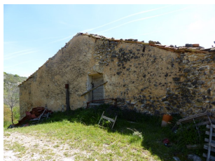
Ensemble oriental. Pignon nord.
