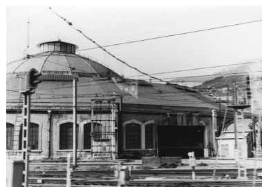
Vue coupole Phot. Dominique Peyre IVR82_20087302012NUC
