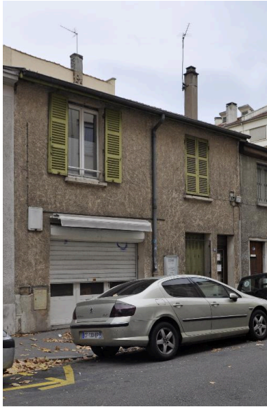
Façade principale Phot. Magali Delavenne IVR84_20166902081NUCA
