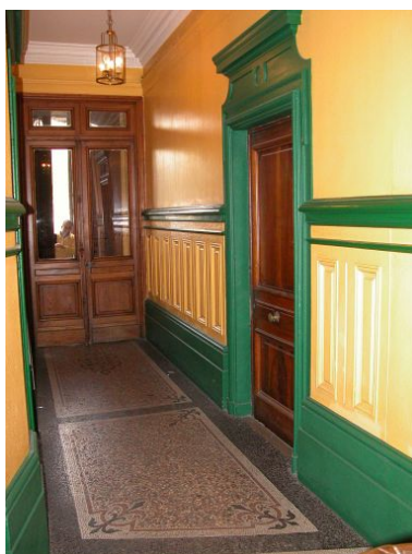
Allée Phot. Phot. Inv. V. Belle IVR82_20046900562NUCA
