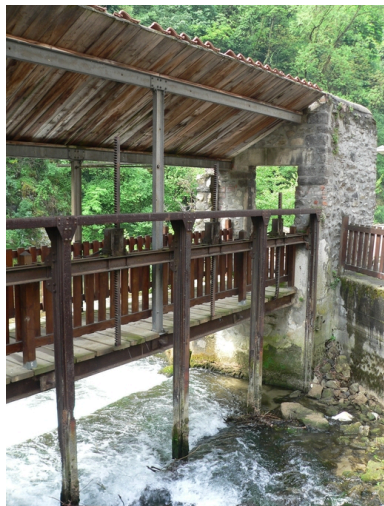
Ecluse Phot. Isabelle Dupuis IVR82_20093800469NUCA
