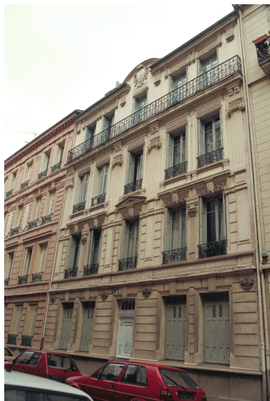
Façade principale Phot. Cendrine Sanquer IVR82_19974202006ZE
