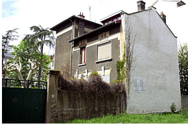
Façade principale Phot. David Chevallier IVR82_20046901048NUCA
