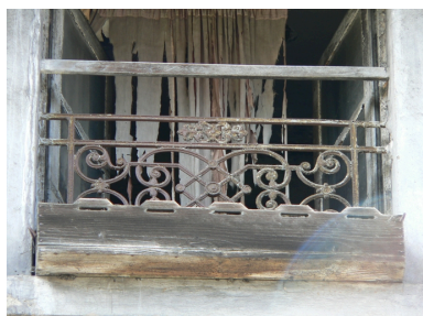
Garde corps Phot. Isabelle Dupuis IVR82_20093800366NUCA
