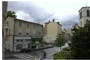
Elévation principale Phot. Maryannick Chalabi IVR82_20106903650NUCA
