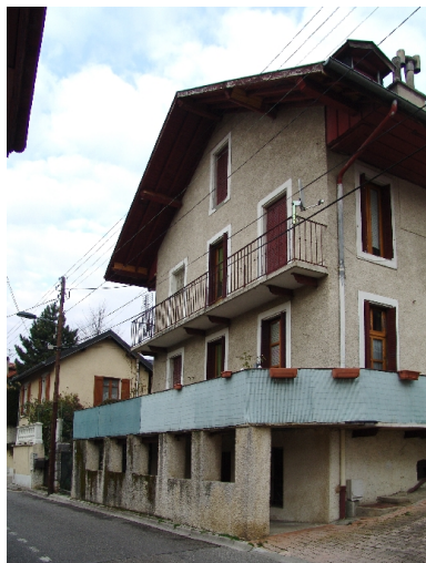
Pignon ouest Phot. François Fouger IVR82_20097300097NUCA
