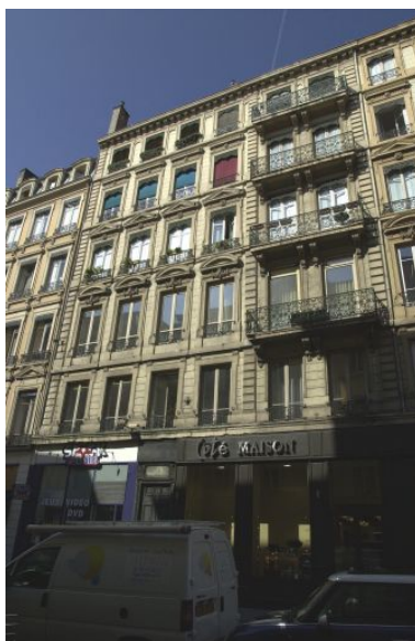
Façade Phot. Bernard Ducouret IVR82_20046905806NUCA
