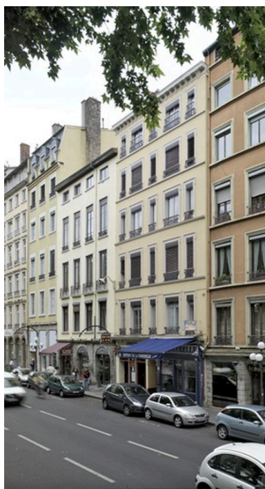
Elévation quai Saint-Antoine Phot. Eric Dessert IVR82_20076902483NUCA
