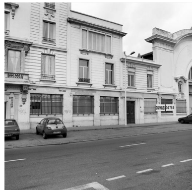
Vue est, façade bureau administration Phot. Martial Couderette IVR82_20016900679X
