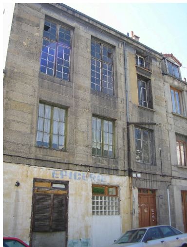
Elévation principale Phot. Cendrine Sanquer IVR82_20084200544NUCA
