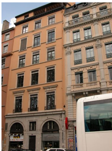
Façade, vue générale Phot. Phot. Inv. V. Belle IVR82_20046900555NUCA
