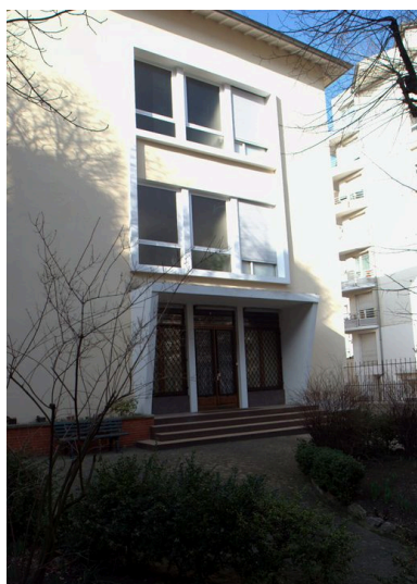
Elévation principale Phot. Maryannick Chalabi IVR82_20106905032NUCA
