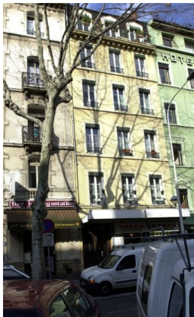
Elévation principale Phot. Maryannick Chalabi IVR82_20016900248NUCA
