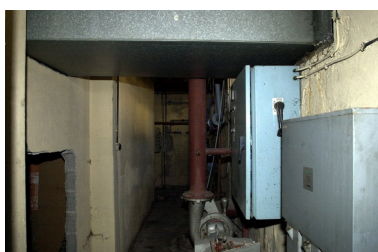
Sous-sol Phot. Nadine Halitim-Dubois IVR82_20036901947NUCA
