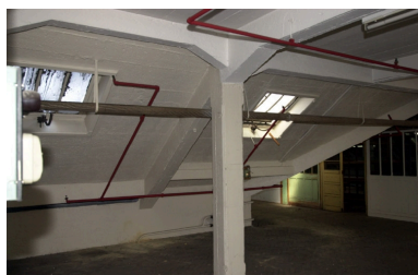
Charpente béton Phot. Nadine Halitim-Dubois IVR82_20036901929NUCA
