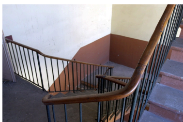
Escalier Phot. Nadine Halitim-Dubois IVR82_20036901944NUCA
