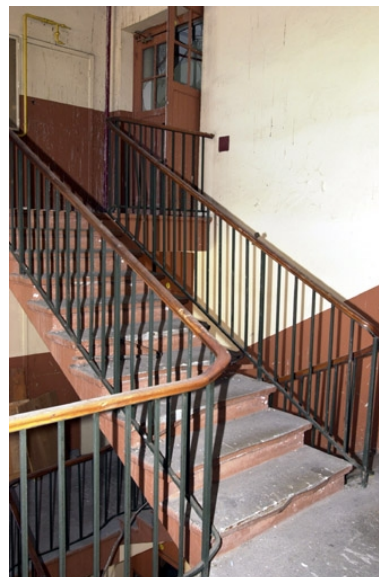
Escalier Phot. Nadine Halitim-Dubois IVR82_20036901928NUCA
