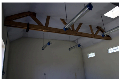
Charpente bois Phot. Nadine Halitim-Dubois IVR82_20036901954NUCA
