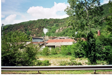
façades sud Phot. Sébastien Durieu IVR82_20042600137NUCA
