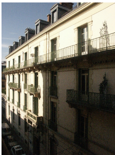
Façade rue Daquin Phot. François Fouger IVR82_20047300093NUCA
