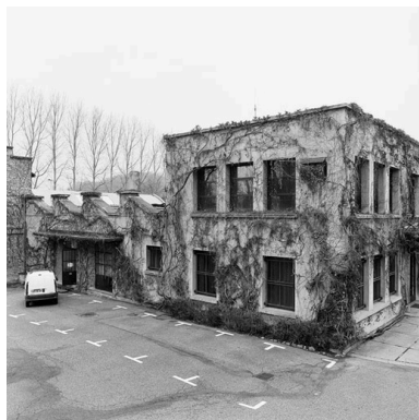
Bureaux et ateliers sheds (1936) Phot. Didier Gourbin IVR82_20043800008X
