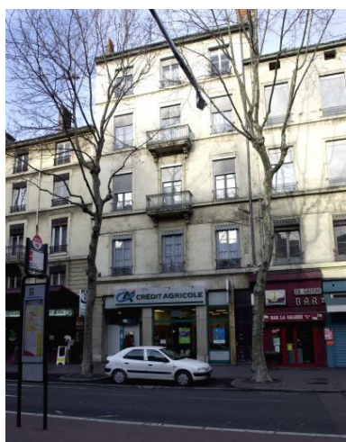
Elévation principale Phot. Maryannick Chalabi IVR82_20016900230NUCA
