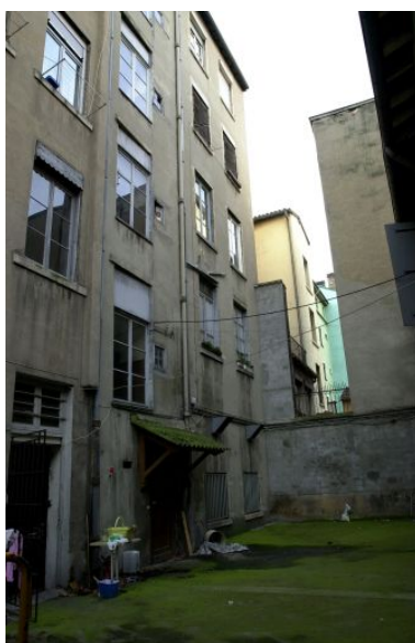
Elévation postérieure Phot. Maryannick Chalabi IVR82_20016900231NUCA
