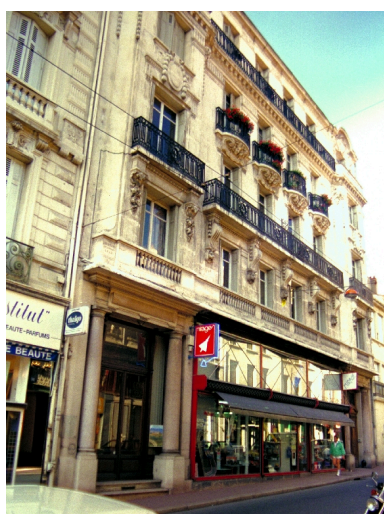
Façade principale Phot. Cendrine Sanquer IVR82_19974202086ZE
