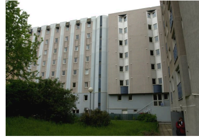
Elévation postérieure Phot. Maryannick Chalabi IVR82_20016902397NUCA
